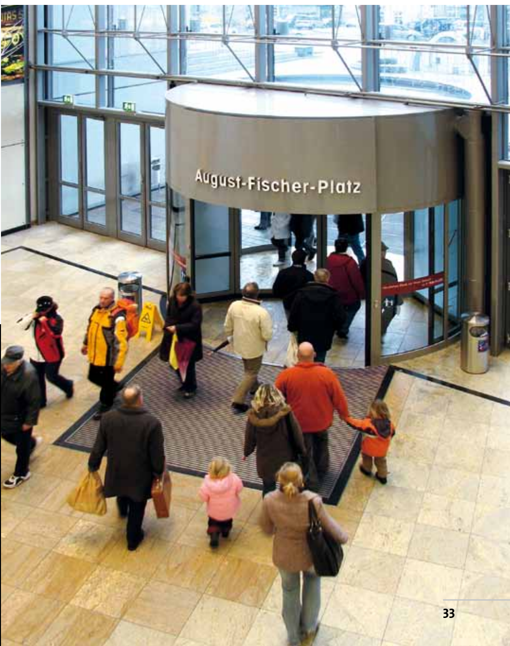
Right: The "Forum Allgäu" shopping centre in Kempten is accessed via very busy revolving doors. With the high-volume spaces and wide corridors inside, this could produce massive draughts of cold air. The RONDO SDA air curtain devices prevent this unpleasant, expensive loss of energy.
