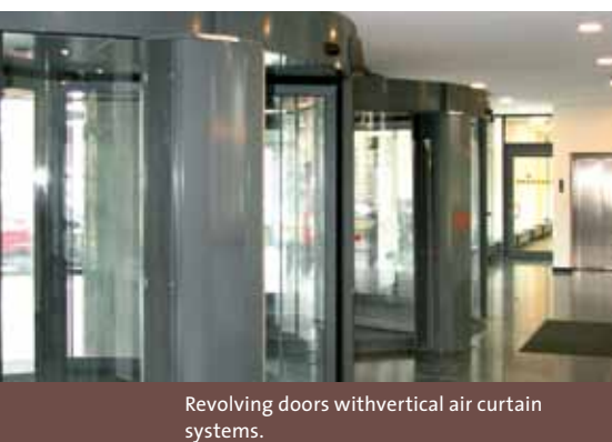
Circular sliding door with vertical air curtain device.
